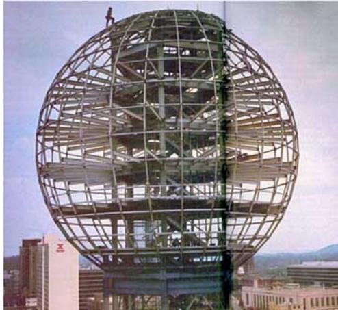
Figure 2: A photo showing the construction of the Sunsphere. Note the 30 curved steel columns and 13 horizontal steel hoops that support the loads of the windows, observation decks, and restaurant. [2]
