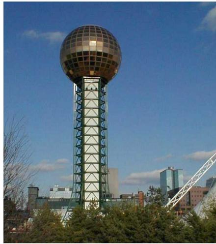
Figure 13: The interior of the Sunsphere has been enclosed to protect the elevators. This picture shows how that reduces the light appearance of the structure.
